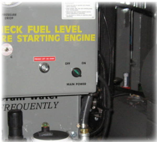
Figure 6: ON/OFF switch for pulse control
