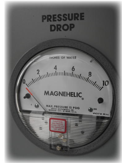
Figure 17: Filter restriction (low if no restriction or clean, high if restricted or dirty) and Pulse power
